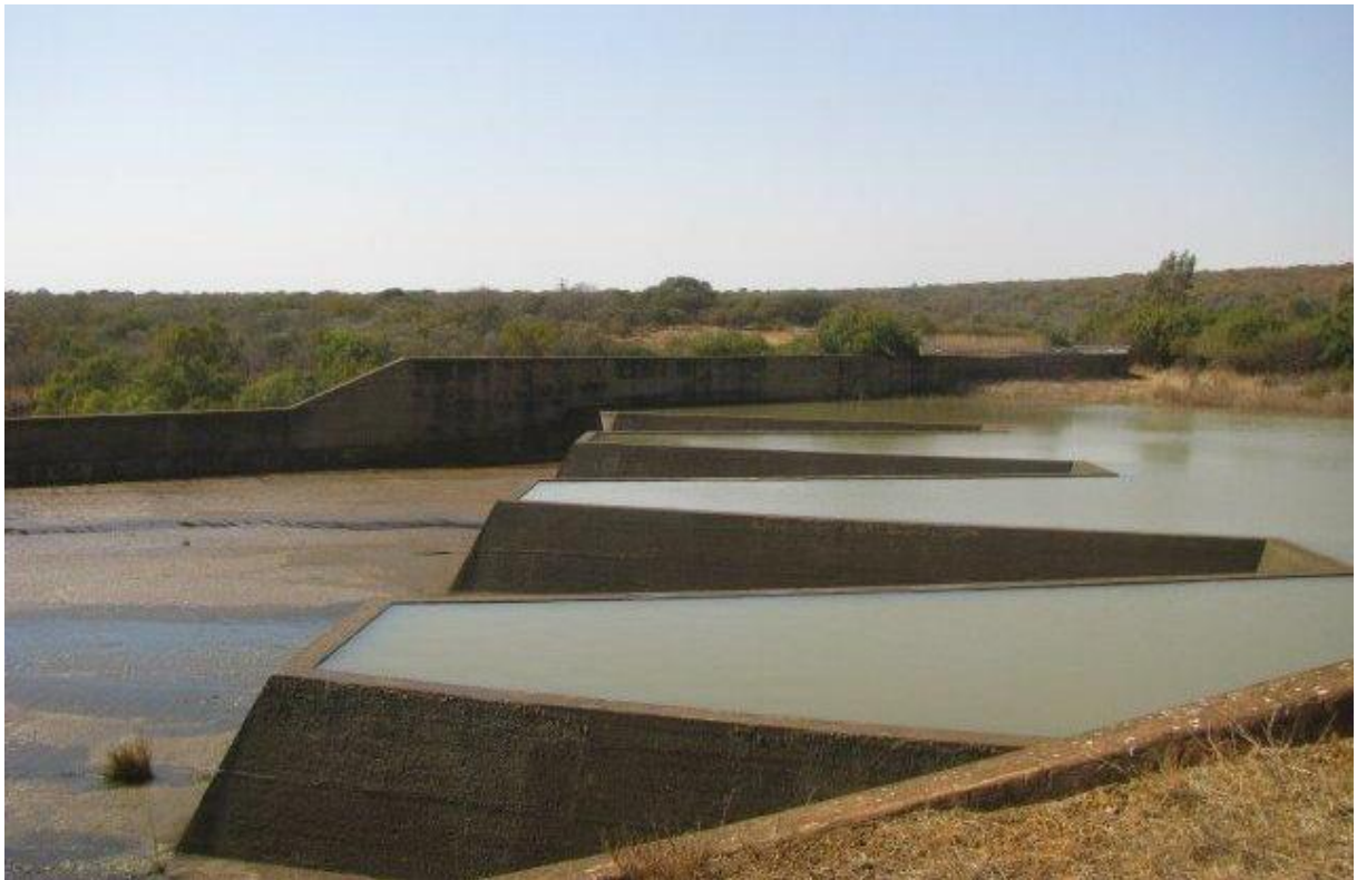
Figure 3-1 Spillway - Marico-Bosveld Dam
